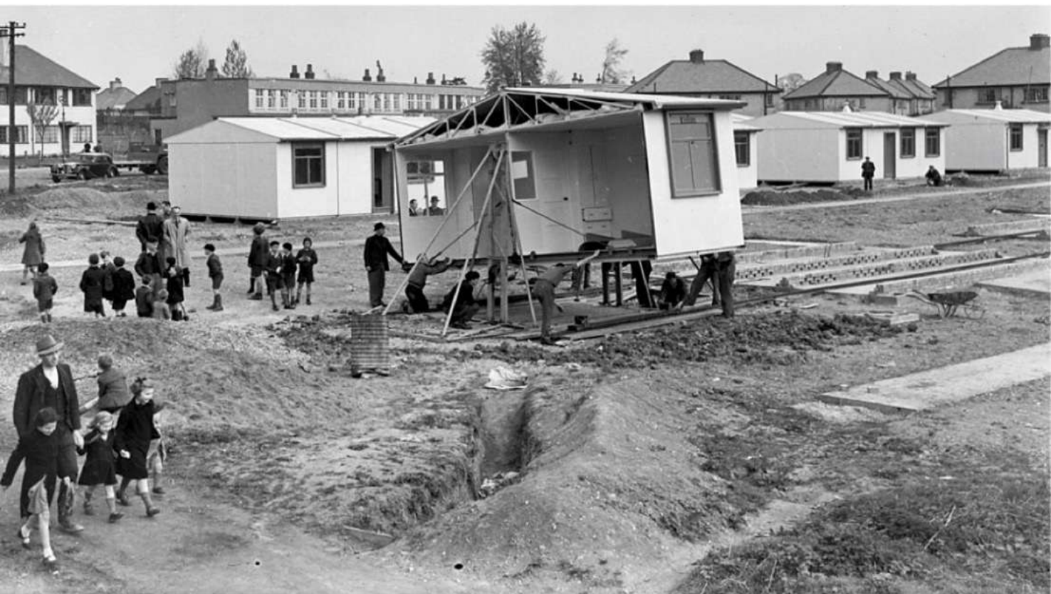
Schoolchildren watch labourers construct a new estate of prefabricated houses in Watford, Hertfordshire, 1946. Photograph: Keystone Features/Getty
